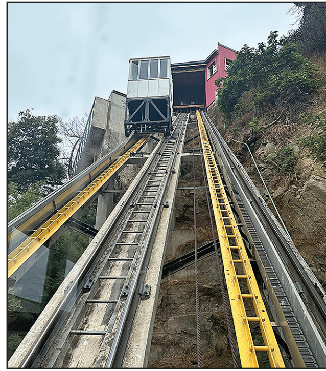
Constructed in 1883, Concepción is the oldest funicular in Valparaíso. Climbing over 225 feet at an angle of 45°, Concepción remains one of the city's most popular ascensors.
